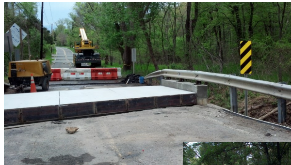
Bridge During Construction
